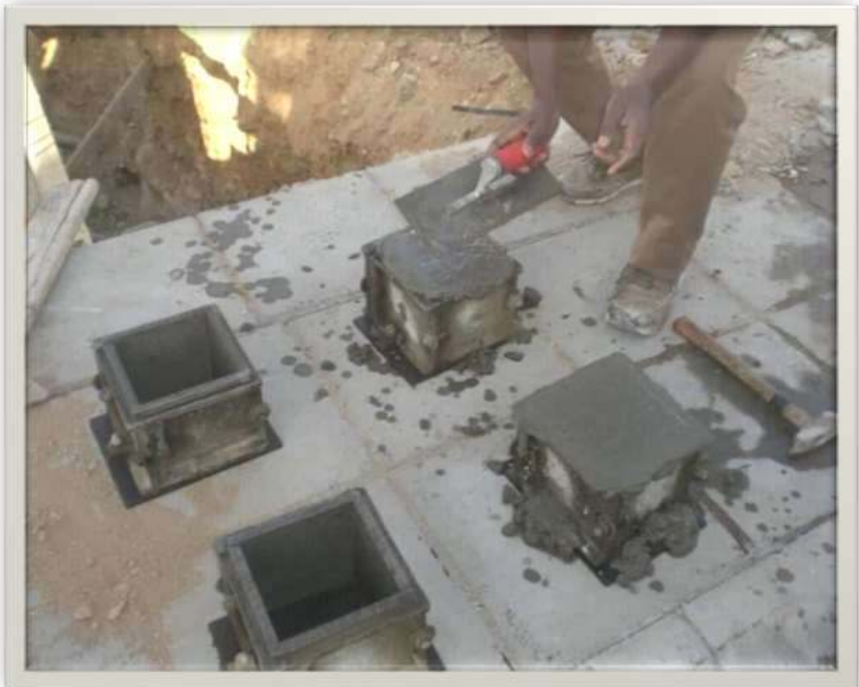
Figure (4) shows the process of pouring blocks and concrete
