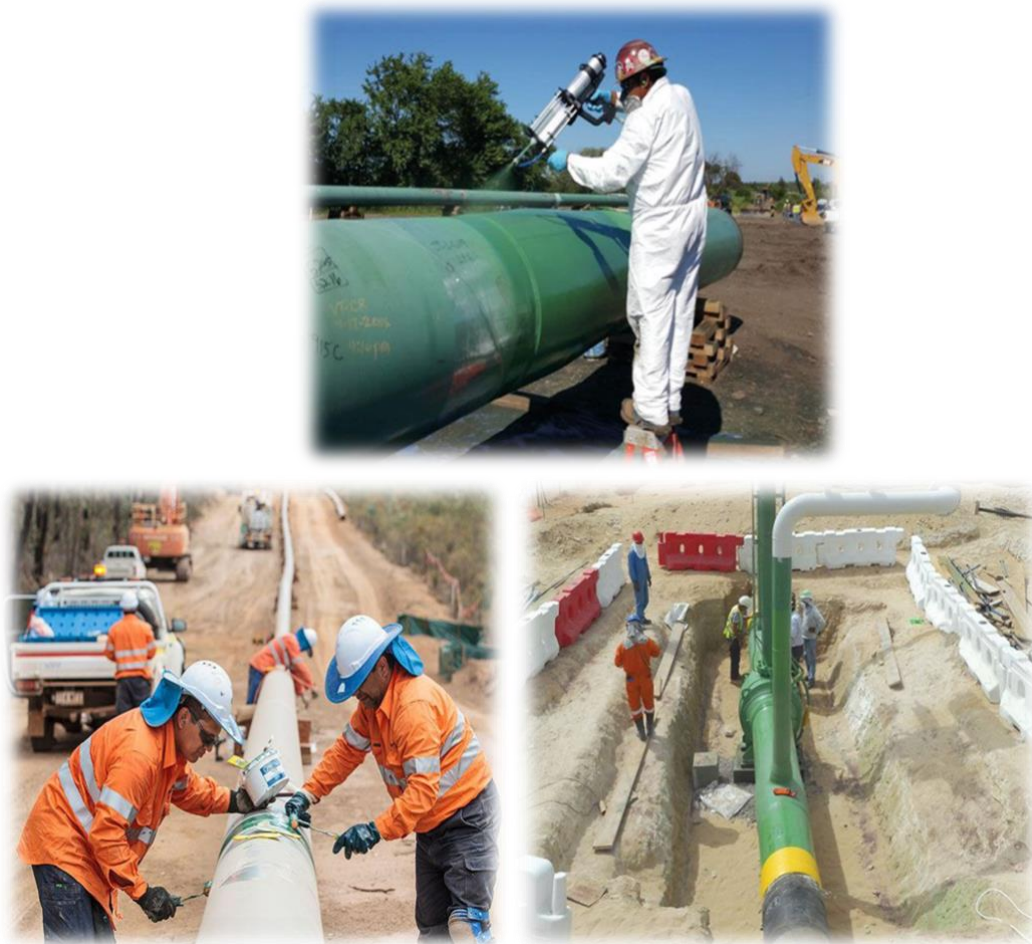
Figure-2.1- Epoxy coating for crude oil pipes
