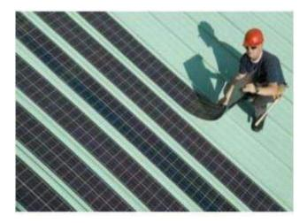
Figure (3-9) CIS thin\_ film
