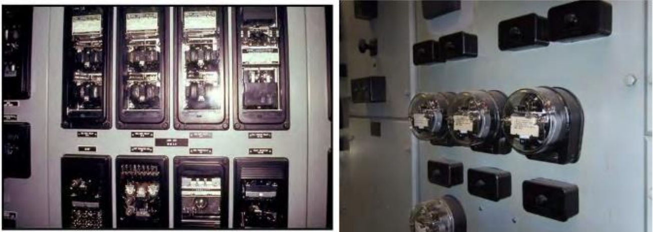
Figure 1.4 Electromechanical Relays
