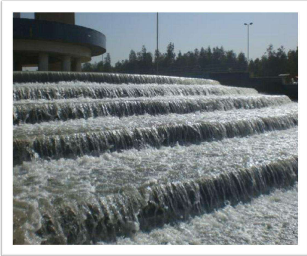
Figure 1.8 Stepped spillway used for recreational purposes at Al-Jadriah Lake, Baghdad, Iraq (Ministry of Water Resources Iraq 2012).
