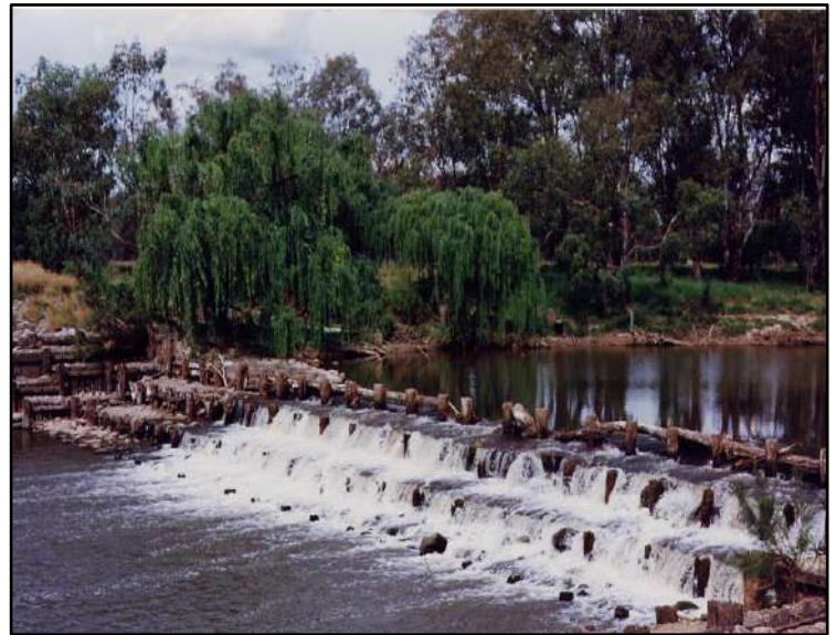
Figure 1.3 Cunningham Weir (Texas, Qld, Australia, 1953; RJW 1999).
