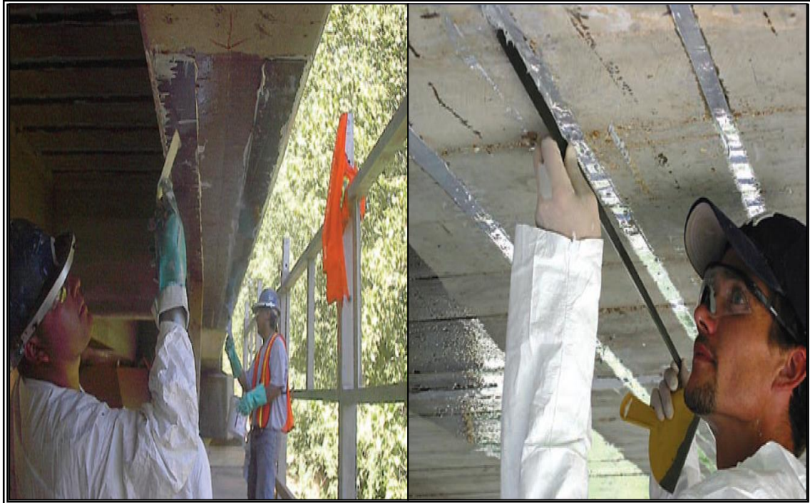
Figure (1.2) FRP Application in a Bridge
