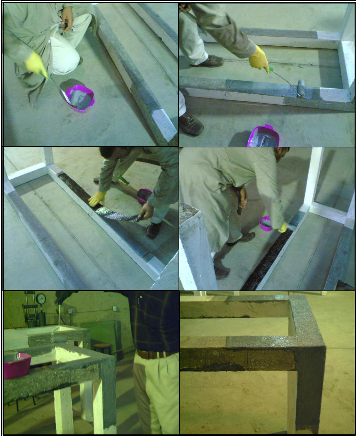
Figure (3.7) Installation of CFRP Strengthening System
