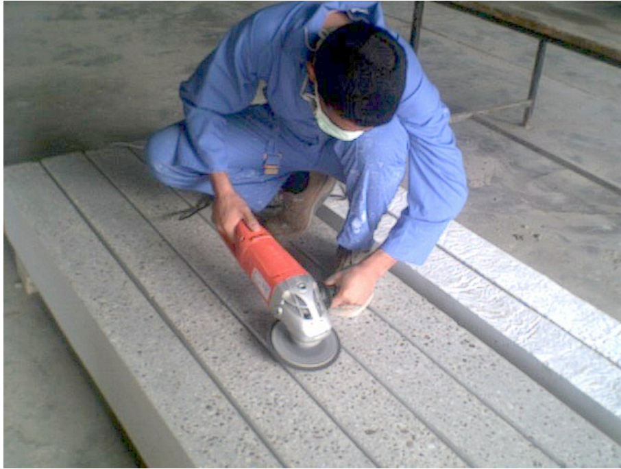
Figure 3.10: Concrete surface preparation by electrical grinder
