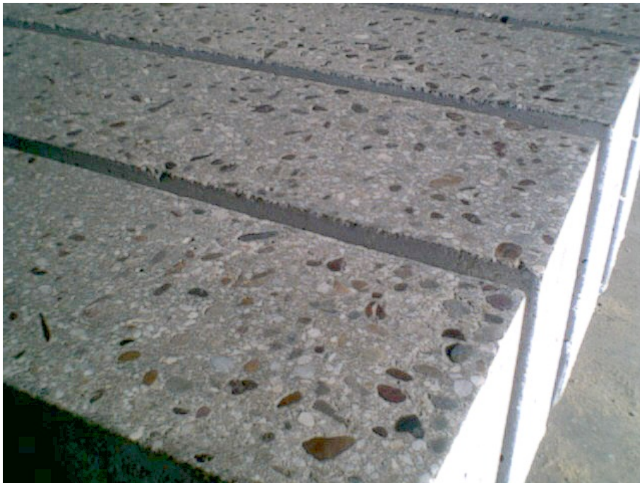
Figure 3.11: Exposed aggregate after surface preparation
