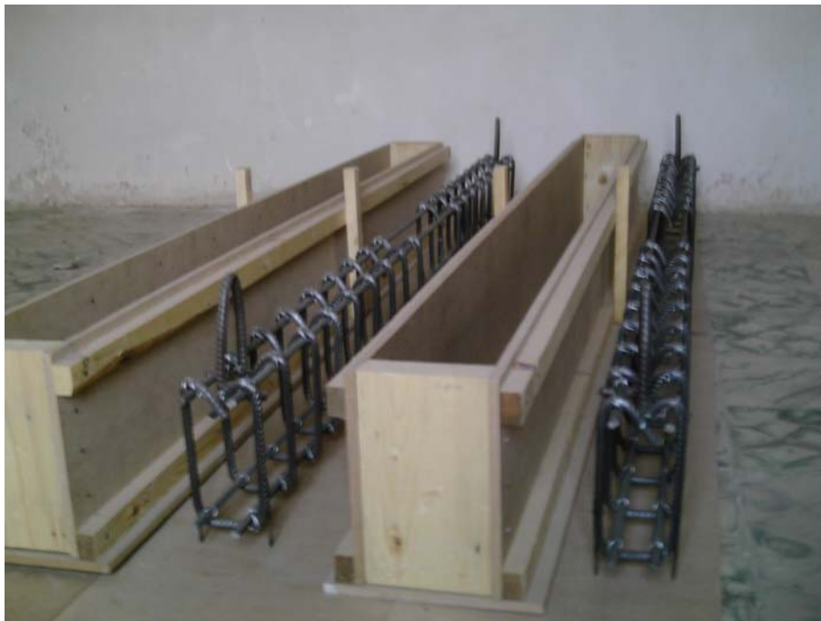
Figure 3.8: Wooden formworks and reinforcing cage
