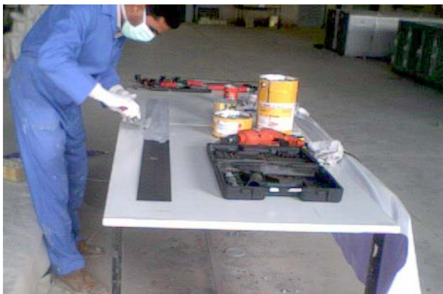
Figure 3.12: Applying epoxy adhesive to CFRP laminates
