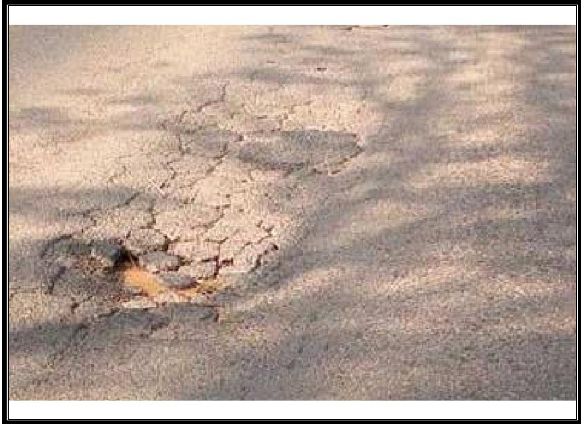
Figure (2-4) Pothole
