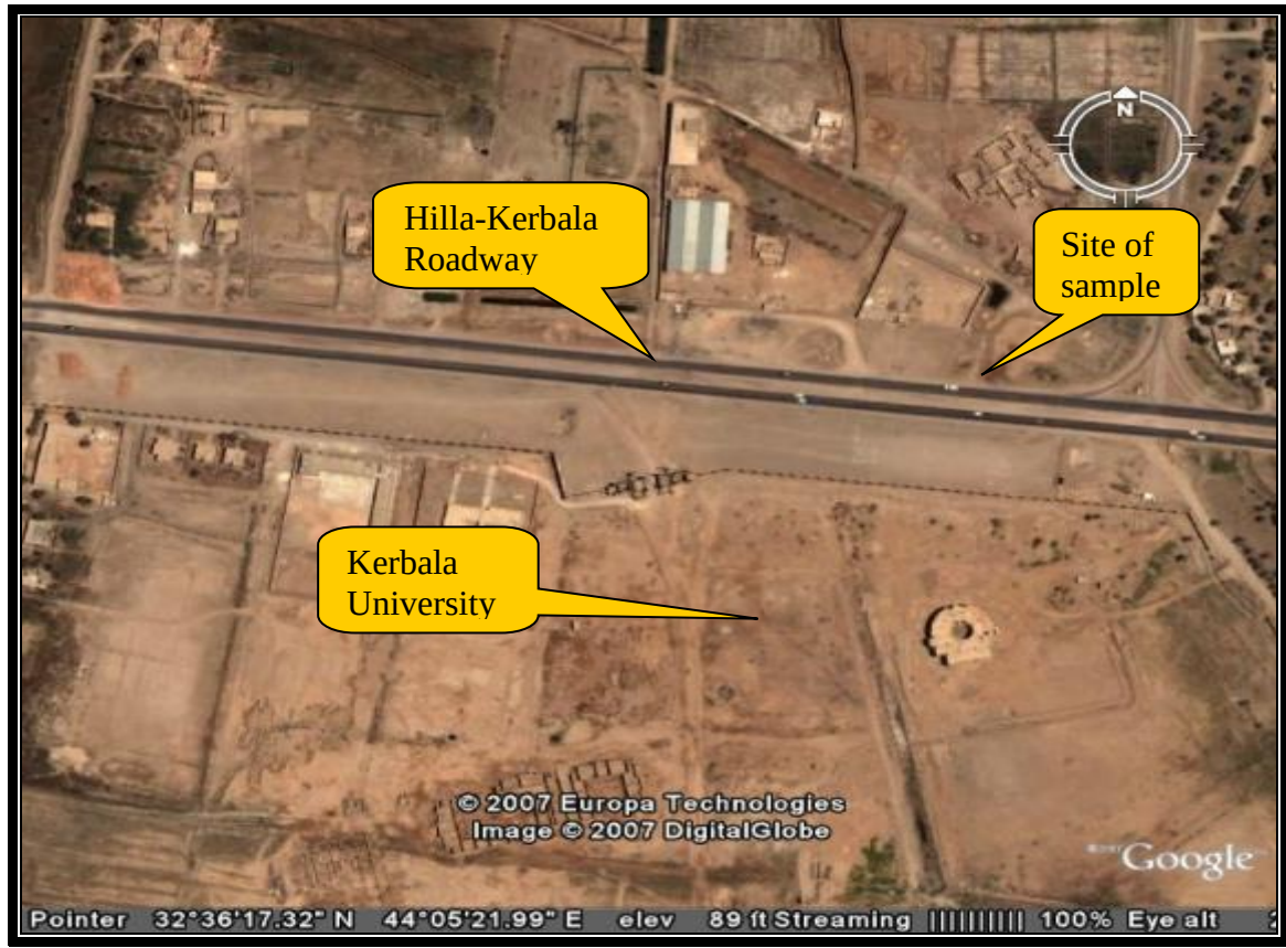
Figure (3- 1) Site View Showing the site of Kerbala-Hilla roadway
