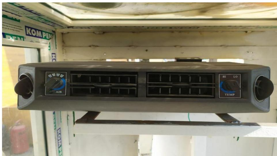
**Figure (3,7) Evaporator and blower unit**
