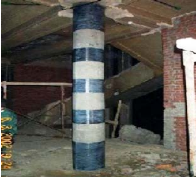
a) Increase axial load in office building [14].
