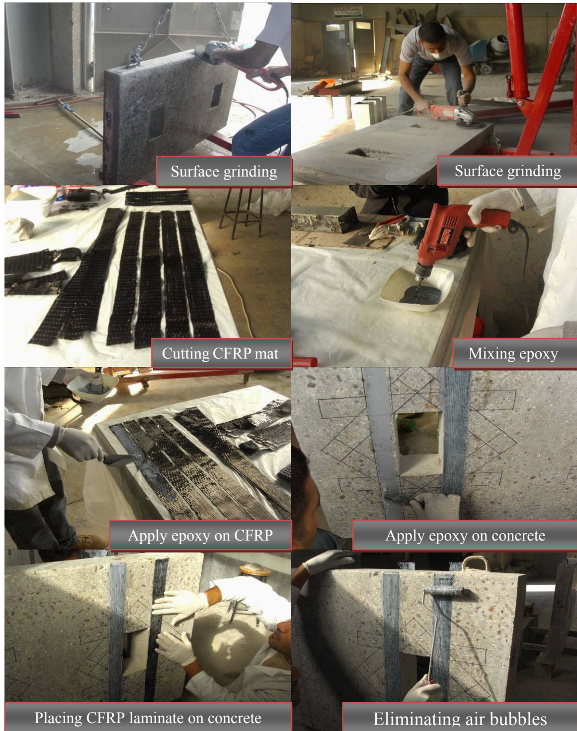
Figure 3.4 application of CFRP system on concrete element
