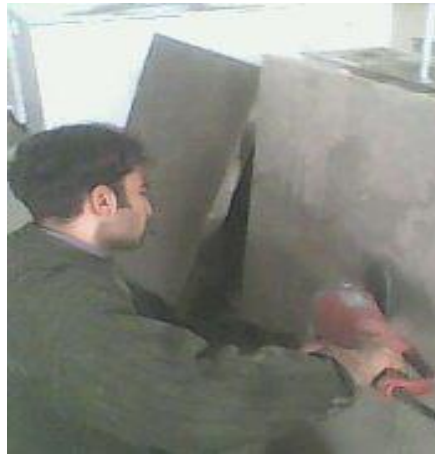
Figure (4-12): Concrete surface preparation by electrical grinder.
