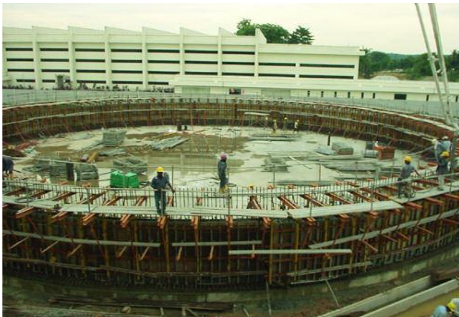
(a) A circular reinforced concrete tank under construction.
