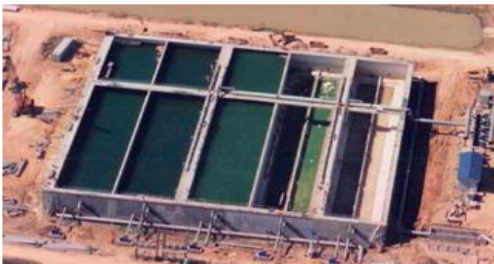
(b) A rectangular reinforced concrete tank under construction.
