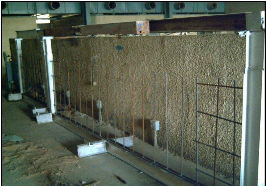
Plate(3-2)Restraining frames of walls of L/H 2 and 4 respectively and their reinforcement
