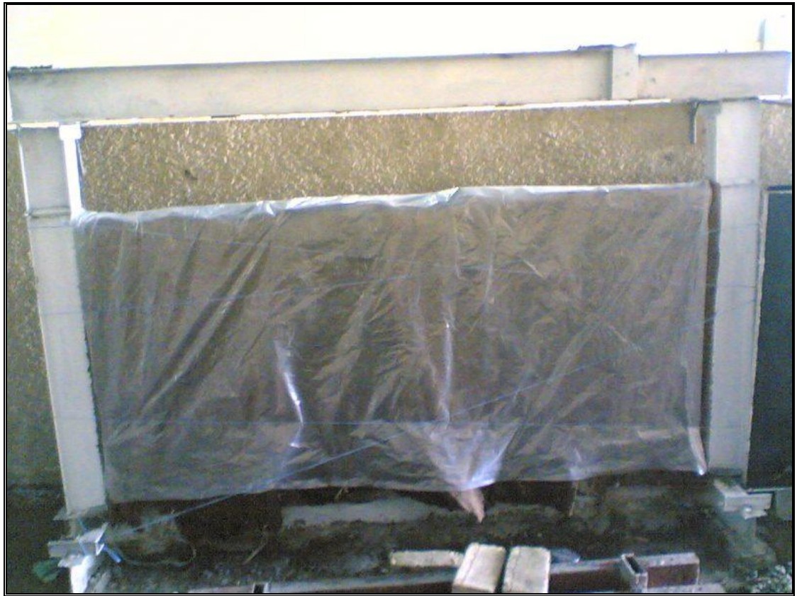
Plate(3-5) Curing of wall (2W)
