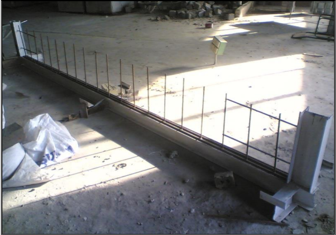
Plate(3-3)Restraining frame of wall of L/H (8) and its reinforcement
