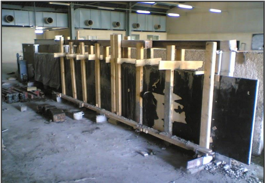
Plate (3-4) Form work of wall (4*1) m
