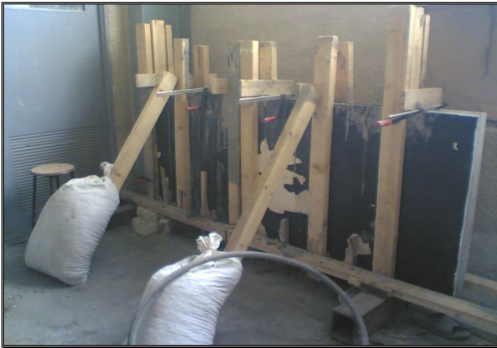
Plate (3-1) Wall formwork.
