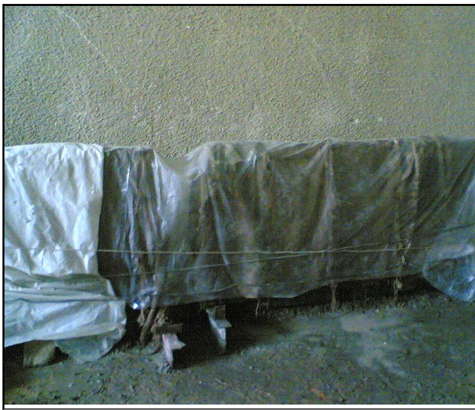
Plate (3-2) Curing Method
