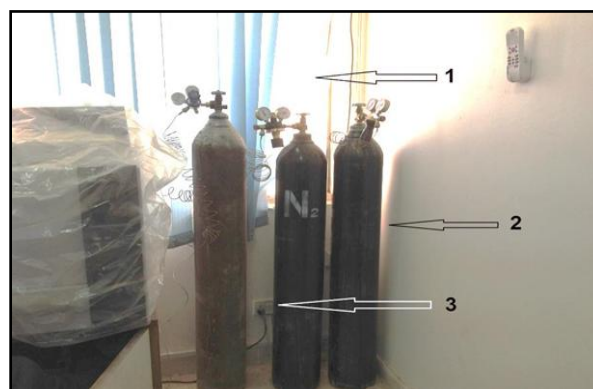
Figure 1. New GC with gas cylinders improperly installed, resulting in a number of safety hazards
