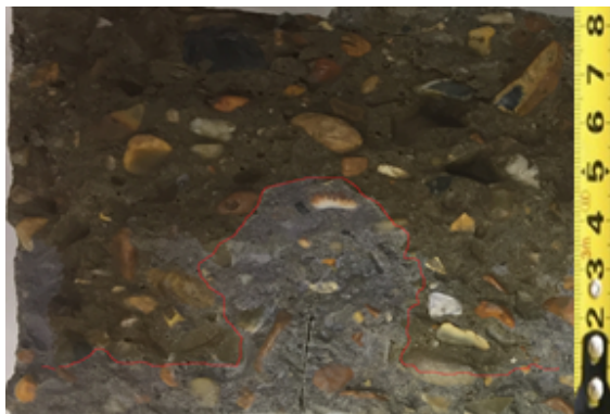
Figure 2: Effect of crack on chloride penetration (M 0.35 with crack width 0.35mm at 30°C)
