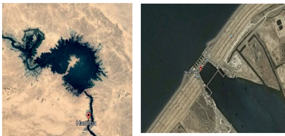
Fig. 1 : Formation of Haditha Reservoir and site plan of the dam region (Google Earth)
