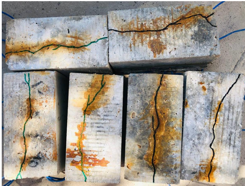
Figure 8: Crack Pattern for Concrete
