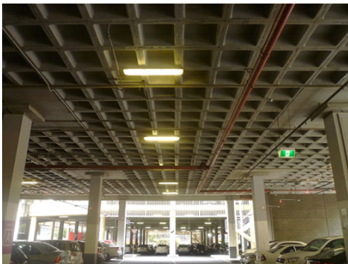
Fig. 1. Waffle slab with opening
