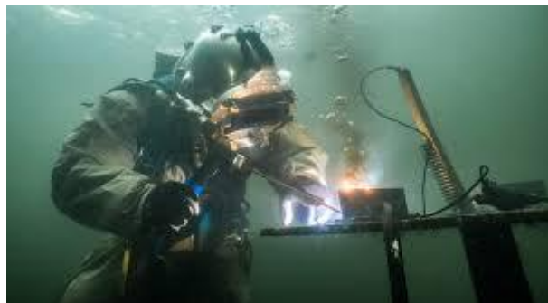
Under water welding(للاطلاع)
